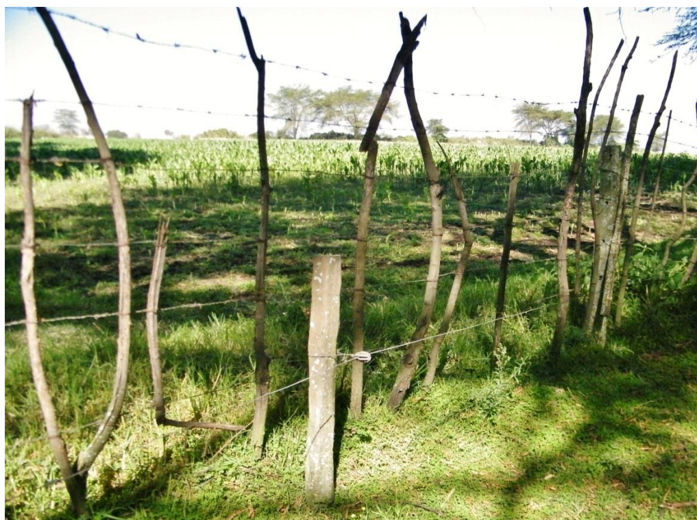
Figure 8: A section of fence constructed to separate wildebeest from cattle. The fence consisted of 3 layers. The main structure consisted of 5ft posts, approx. 10ft apart, joined by four lengths of barbed wire. Bamboo poles were then strung vertically to give the fence height, which could be easily seen by wildlife. An electric fence ran around the outside of the main structure, approximately one metre from it. The electric fence consisted of four wires strung between 3ft high wooden posts. Finally, there was a fence running internal to the main structure, this time five metres out to prevent cattle-wildebeest contact. This internal fence was 3ft high, with a single electrified wire and wooden posts – this wire was moved depending on the grazing fields in use.
